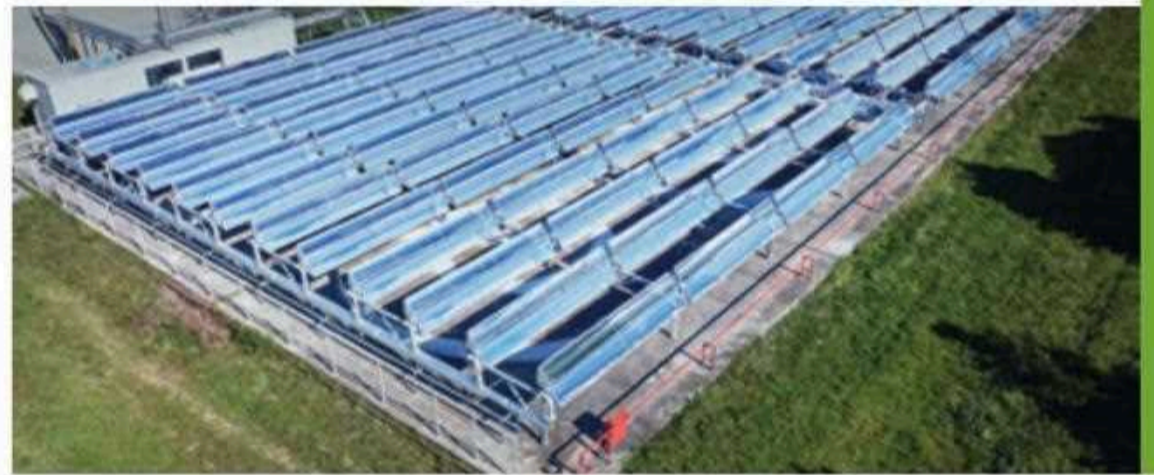
Parabolic trough collectors for one of the breweries of the Carlsberg Group in Salonika, Greece Photo: Absolicon
