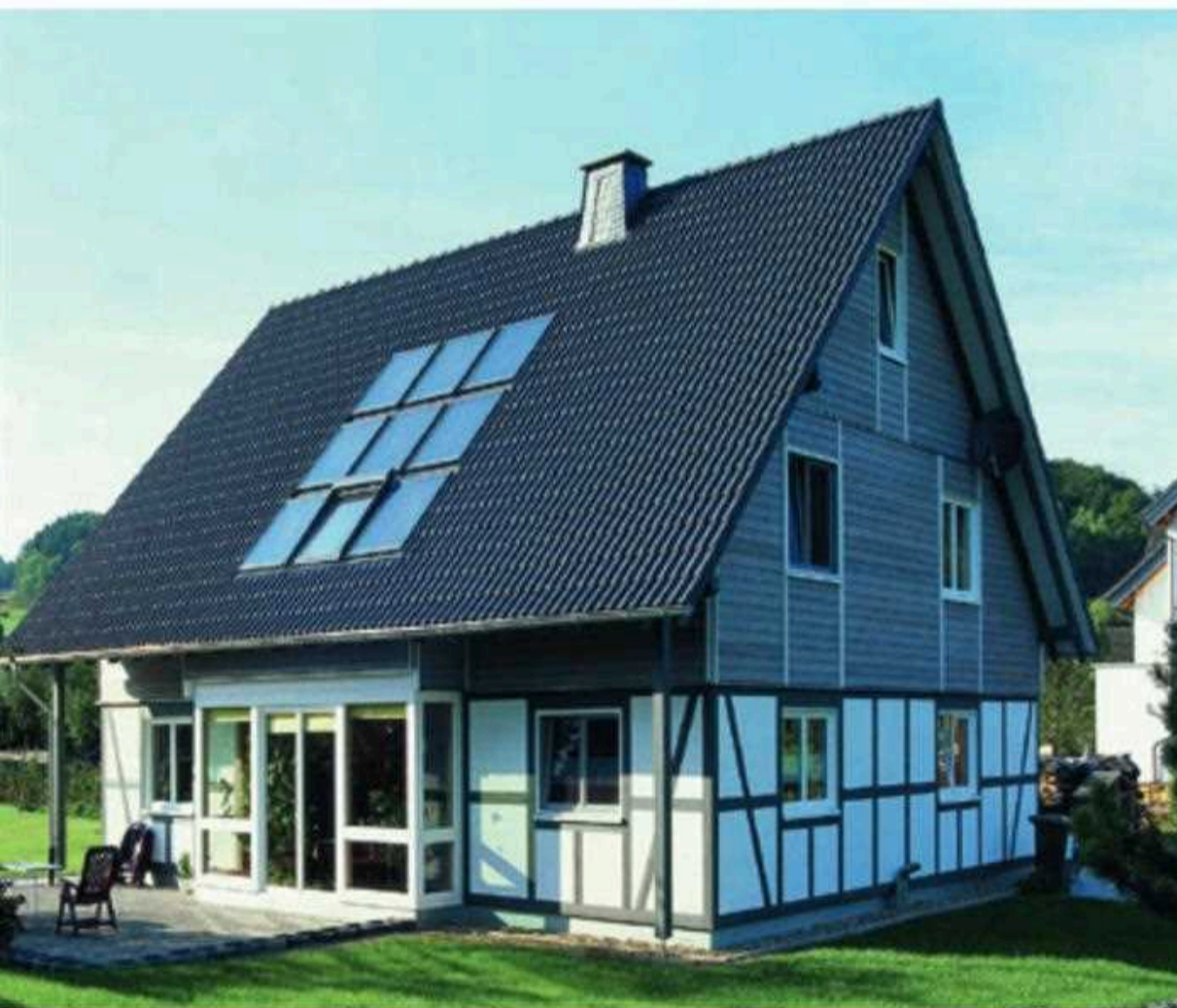
Roof-integrated solar system for hot water preparation Photo: Velux / Solar Heat Europe
