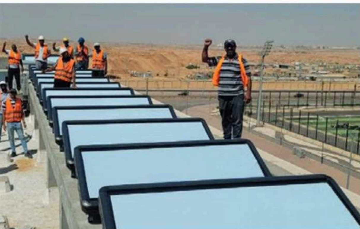
Installation of Sunpad systems in Cairo, Egypt Photo: GREENoneTEC Solarindustrie GmbH, Austria
